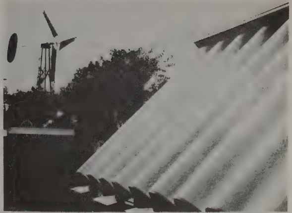
Exterior of Test Model for Cape Cod Ark. Panels of Kalwall are arched for more effective solar trapping. Design by Solsearch Architects.
